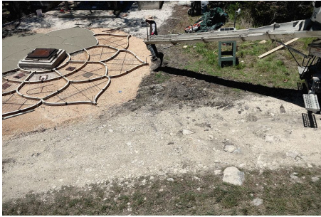
Nine cubic yards by chute: the truck at the edge of the site, the chute over the forms.
