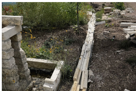
Laying the limestone rill by hand.
