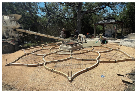
Pour day at ground level: the chute over the forms, the crew at the plinth, the shrine behind.
