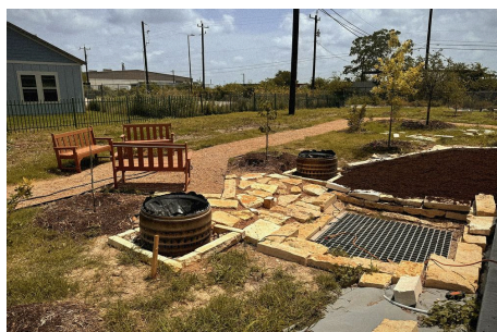
The court laid, before planting.
