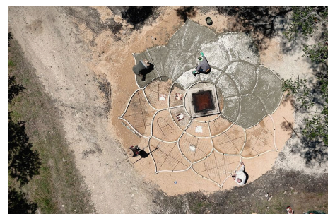
Half poured, from straight above: birch forms on one side, fresh concrete on the other.
