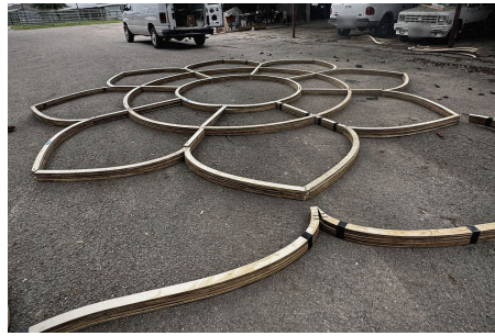
The eight petal forms laid out dry on the yard to check the figure before the haul.
