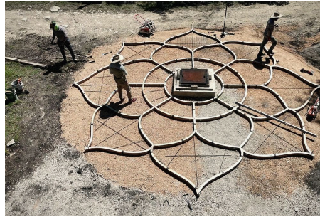
The forms set on the prepared ground: one family of laminated birch ribs to each petal, the mesh going in.
