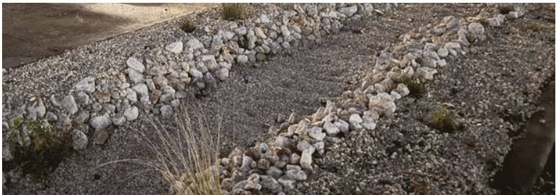
Curbside bioswale, Alamo Heights. · In service since 2025.
